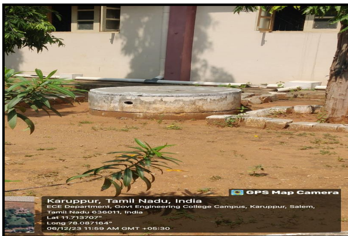
Figure 1: Rainwater harvesting Pit in Department of ECE
